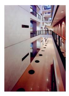
Mass has therefore been used here towards sustainability. It resulted in a building without air conditioning and active cooling, so that stale air is discharged via natural updraft in the atrium through six large shafts.
