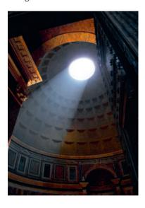
An oculus (an eyelike opening) at the top of the dome is the only source of daylight penetration, and rainwater simply runs off the gently sloping marble floor below. Since the human eye cannot take in the resulting spatial form of the interior at a glance, the space surprises visitors upon entering thanks to a sequence of light-and-dark experiences that encourage movement through the interior to take in the whole building. That is why the interior leaves an indelible impression on the visitor.
